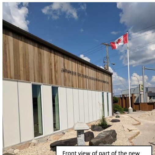
Front view of part of the new expanded Japanese Garden, outside portion (still under construction)
